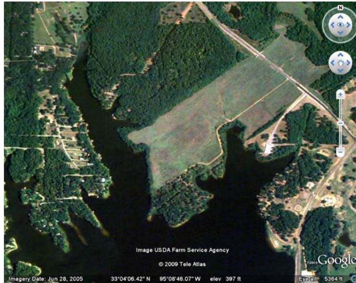
Photo 12: Aerial view of the emergency spillway.
